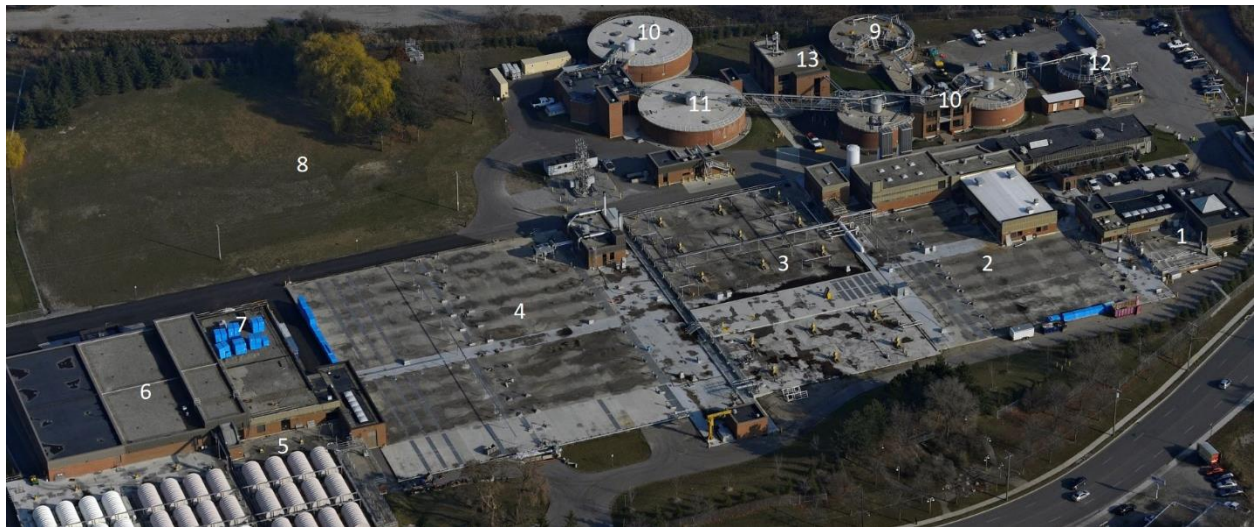
Figure 2.7: Barrie wastewater treatment plant layout 2017: 1 – Pump house, 2 – Primary clarifiers, 3 – Aeration tanks, 4 – Secondary clarifiers, 5 – Rotating biological contactors, 6 – Sand filter, 7 – UV treatment, 8 – Clean water discharge piping, 9 – Aerobic digester, 10 – Primary digesters, 11 – Secondary digester, 12 – Biosolid holding tank, 13 – Co-generation facility (City of Barrie, 2004)
